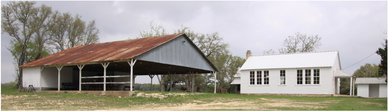
Figure 1: Rheingold School Pavilion & Schoolhouse (Shacklette, 2016)
